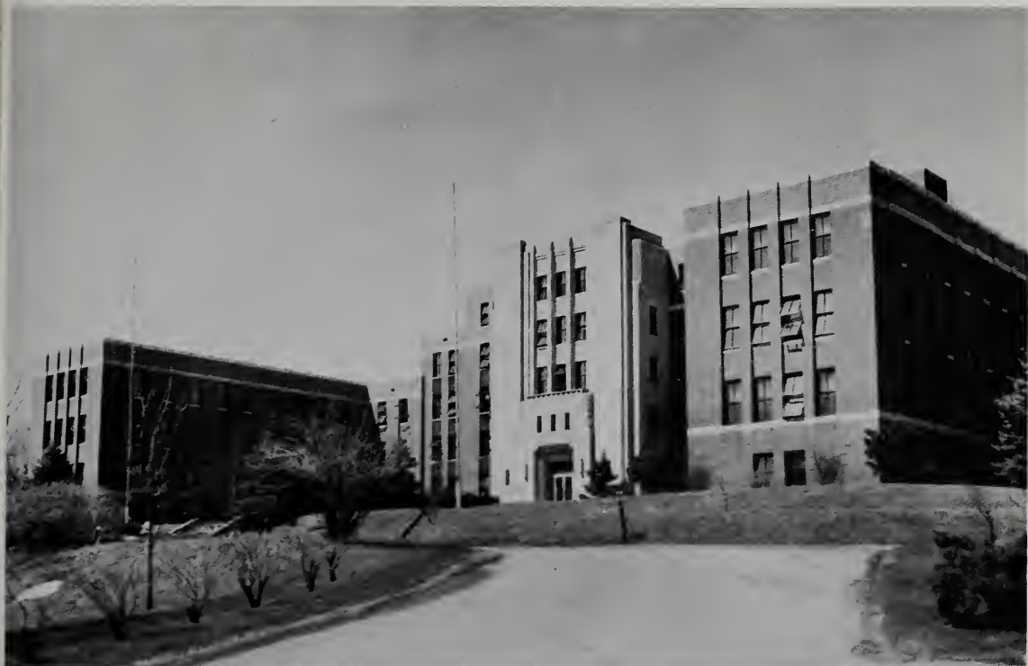
Administration Building, Undercliff Hospital
